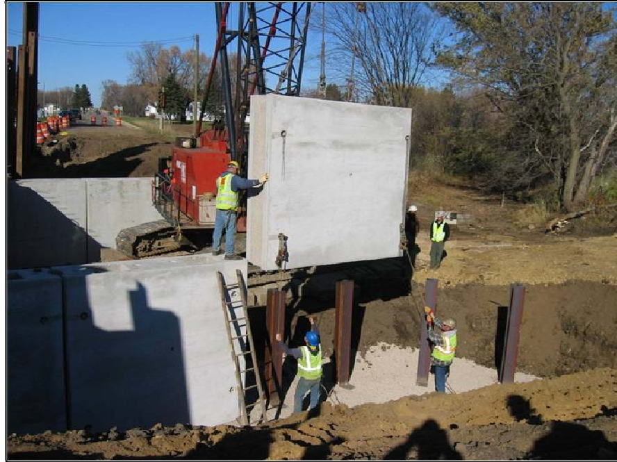
Figure 7.1-2 Prefabricated Abutment
