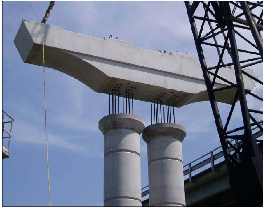
Figure 7.1-1 Prefabricated Pier Cap
