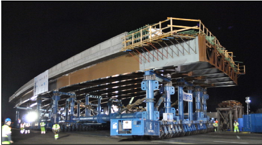
Figure 7.1-7 Self Propelled Modular Transporters Moving a Bridge
