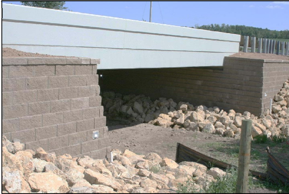
Figure 7.1-4 GRS-IBS Structure
