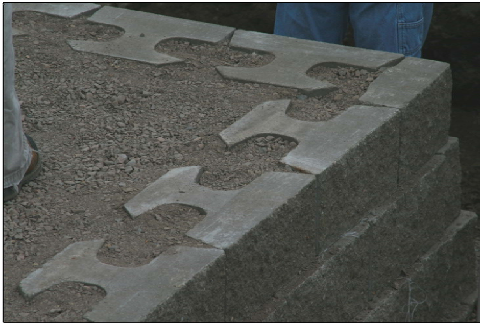
Figure 7.1-5 GRS Abutment Layer During Construction
