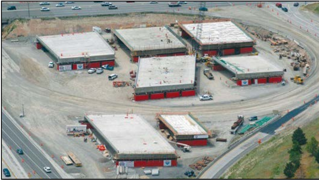
Figure 7.1-8 Example Bridge Staging Area (BSA)
