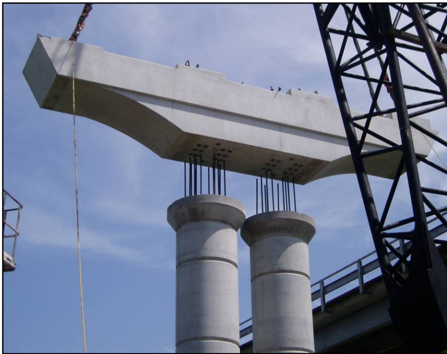
Figure 7.1-1 Prefabricated Pier Cap
