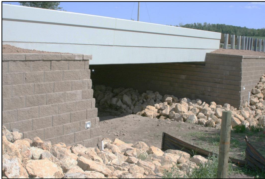
Figure 7.1-4 GRS-IBS Structure
