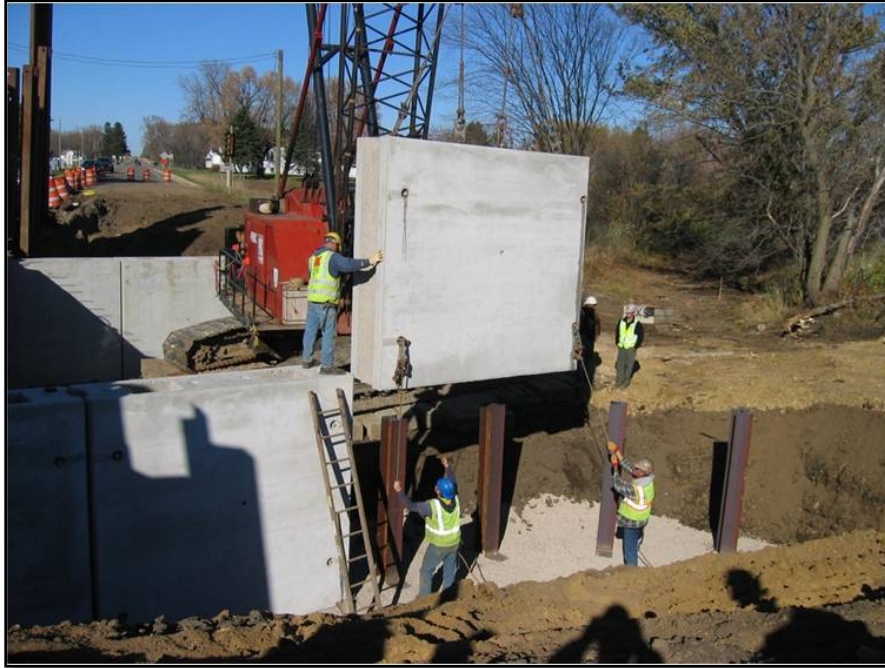
Figure 7.1-2 Prefabricated Abutment
