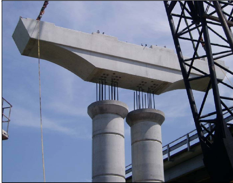
Figure 7.1-1 Prefabricated Pier Cap
