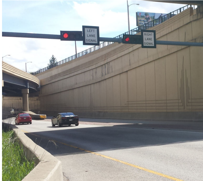
Figure 3.3.3 Lane Designation Signs
