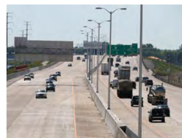
New I-41 Causeway and Bridge.
