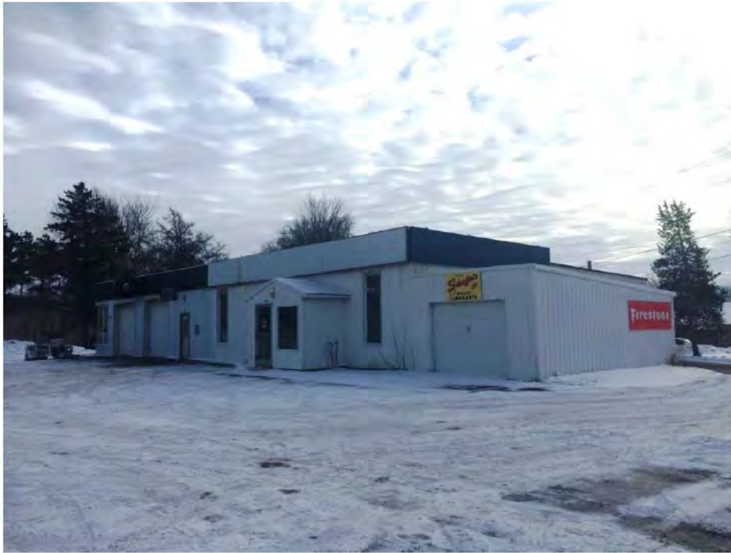
This view looks southeast exhibiting another close up of the subject's commercial building. The additional cold storage area attached to the west end of the building is seen here.
