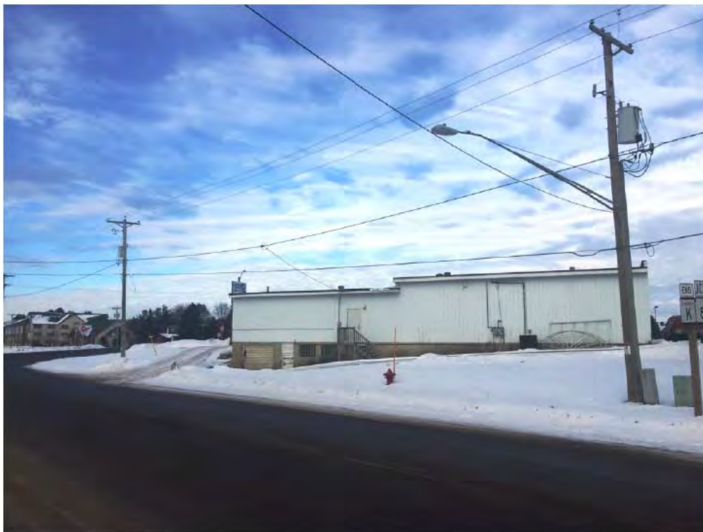
This view looks north at the subject's south side of the commercial building exhibiting an exterior entrance at the rear of the building.
