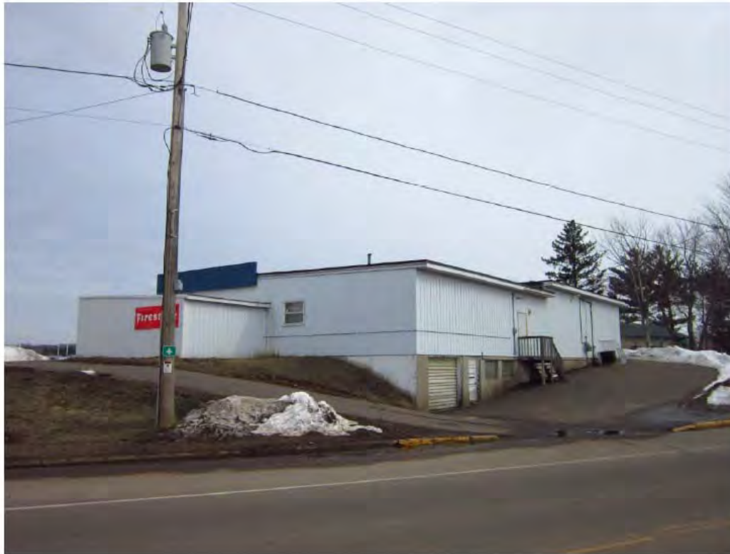
This view looks northeast exhibiting the rear view of the subject's commercial building, secondary access is provided here.
