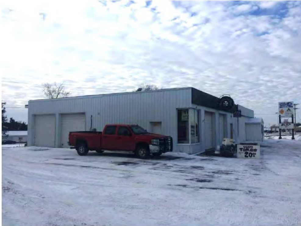
This photo exhibits the subject's commercial building with three entry doors and four overhead service doors.
