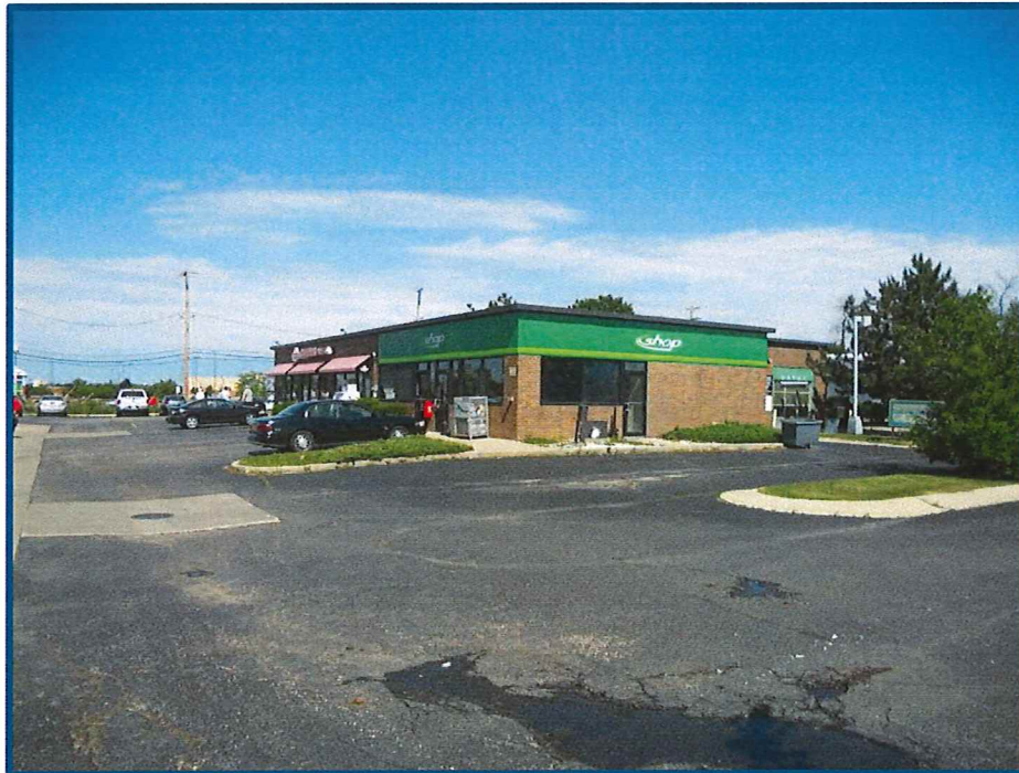
C-Store and Toppers east elevation
