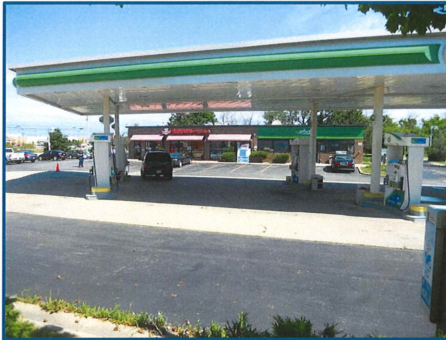
South elevation from STH 50
