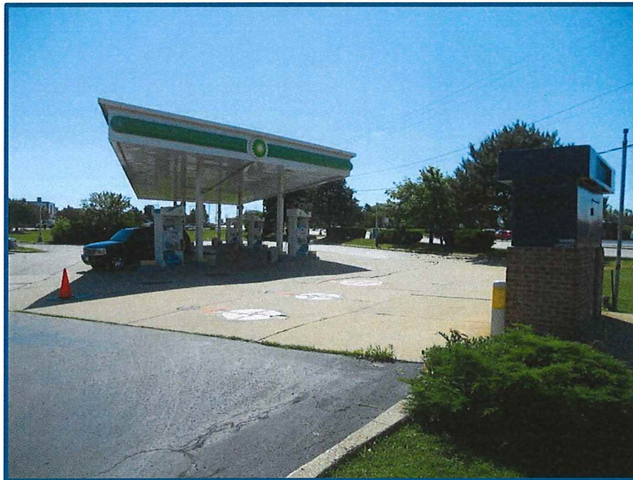
Below ground tanks and canopy/pumps (all being acquired)
