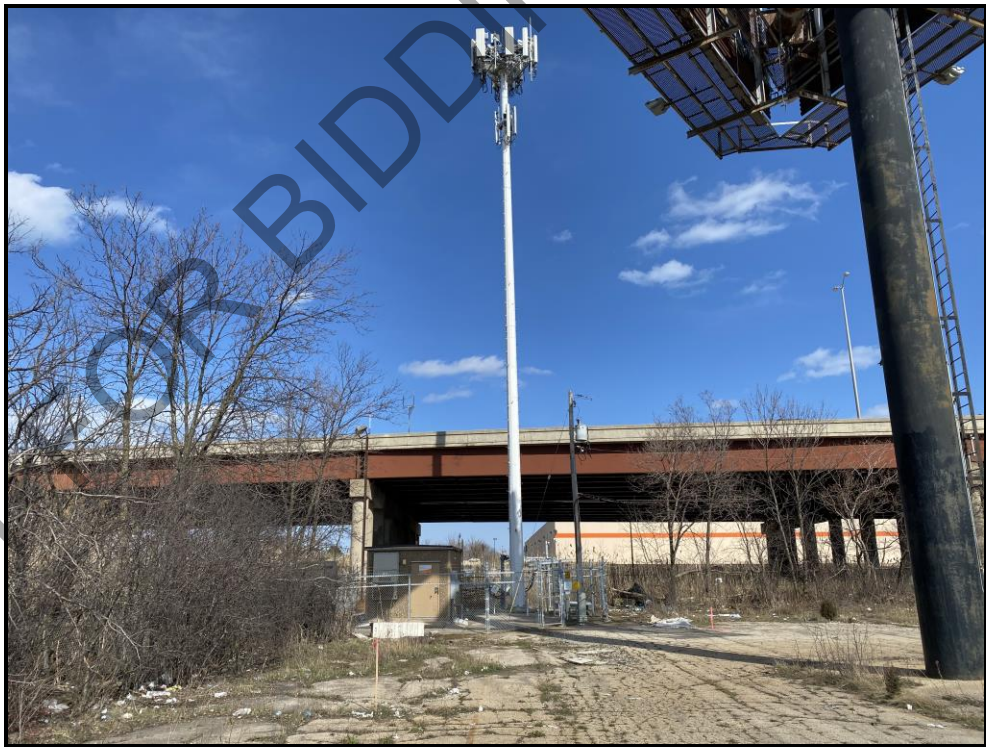
VIEW FACING EAST AT NORTHERN CELL TOWER SITE
