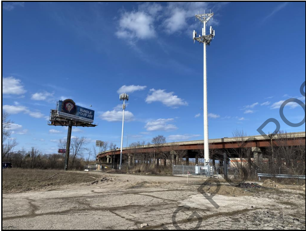
VIEW FACING NORTHEAST AT AREA OF TAKING WITH CELL TOWERS & BILLBOARD
